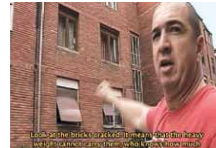
Look at the bricks cracked. It means that the heavy weight cannot carry them, who knows how much. . .
