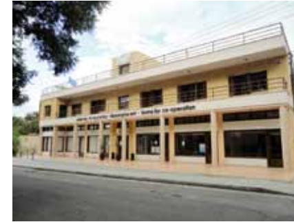
The building at works completion, May 2011.
