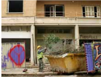
Workers cleaning and preparing the building site, February 2010.
