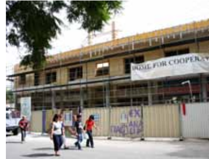
Works in progress six months before inauguration, October 2010.
