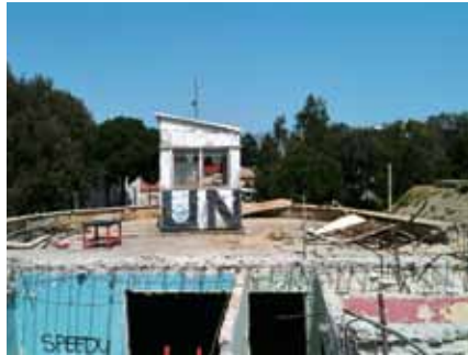
Partial demolition of the roof, April 2010.
