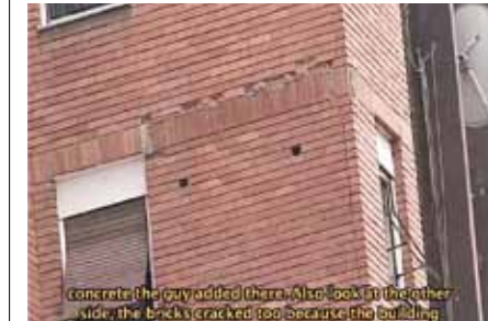
... concrete the guy added there. Also look at the other side, the bricks cracked too because the building. . .
