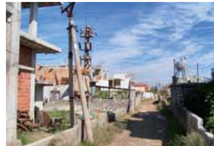
Although the Keneta neighborhood (formerly a swamp in the Adriatic coastal city of Durrës, Albania) is built on a regular land division, drainage canals were the basis for the subdivision of the land, so a serious lack of the most basic communal standards (water, sewage, and electricity) makes housing conditions barely livable.
