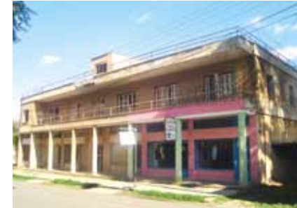
View of the building during first project steps, June 2006.
