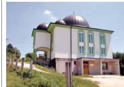
Gornji Ahmići Mosque in the process of rebuilding
