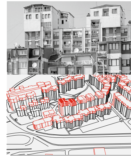
Urban parasites (extensions, annexes, roof extensions and cuts into buildings; houses on roofs). Individual developments; the owners are part of the neighborhood community.
